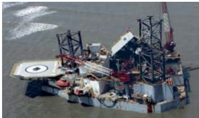
Hurricane Katrina: The Ocean Warwick oil rig was severely damaged by Katrina and drifted a good 100 km from its original position; it went aground on Dauphin Island in Alabama.
