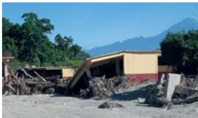
Hurricane Stan: Stan and Wilma caused enormous damage mainly on the Gulf of Mexico, but also in other areas in Mexico. Catastrophic floods reached as far as the Pacific coast. The photo shows a school in Tapachula, Chiapas, destroyed in Hurricane Stan.
