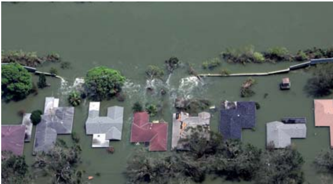
Levee breach on the west side of London Avenue Canal, New Orleans
