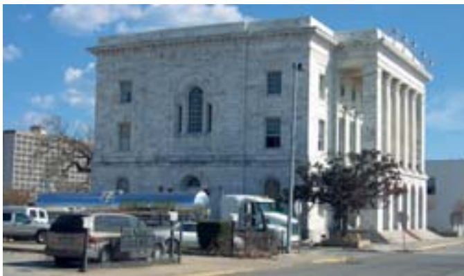
Hurricane Katrina: The City Hall at Biloxi is a sturdily built structure. It withstood the high wind speeds almost unscathed.
