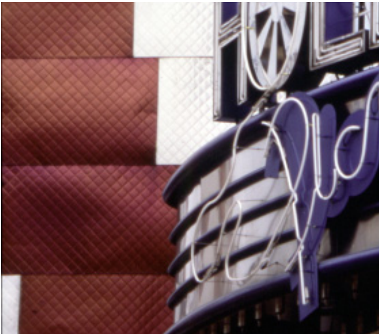
Euro Disney, near Paris, France, makes extensive use of coloured and textured stainless steel eg column cladding and roofing.
