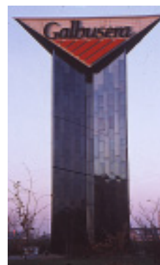
The logo of a confectionary company, at Agrate Brianza (Milan), Italy, is supported by a 22 m high tower clad with electrolytically coloured stainless steel.
